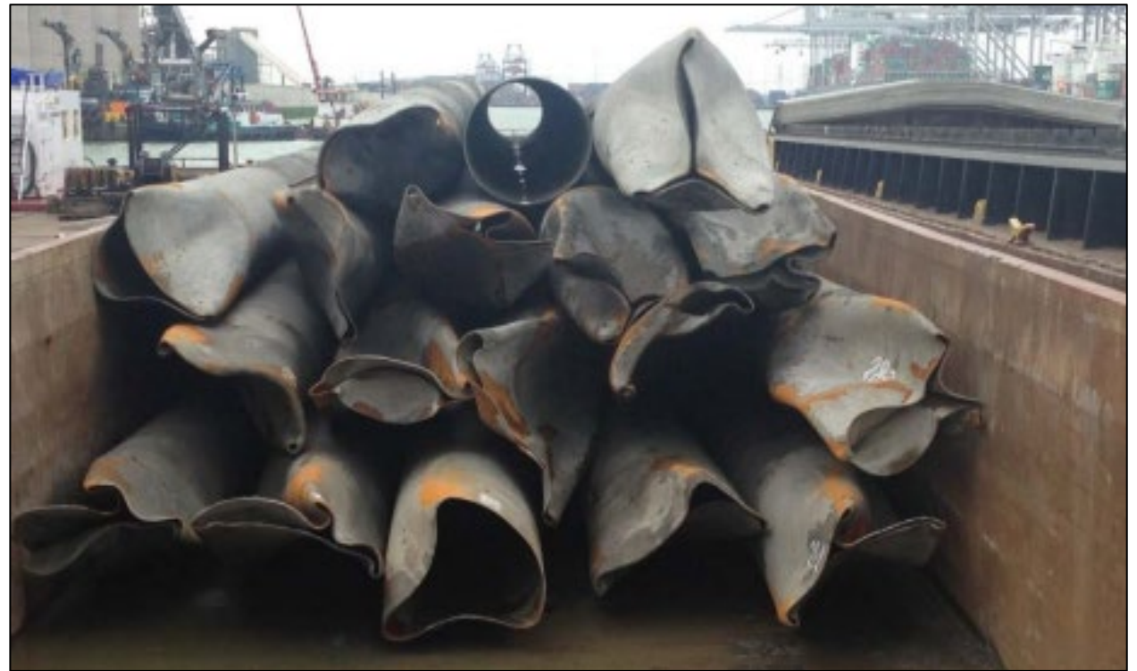
Steel tubular king piles toes heavily damaged during driving for an offshore construction project in Rotterdam.
