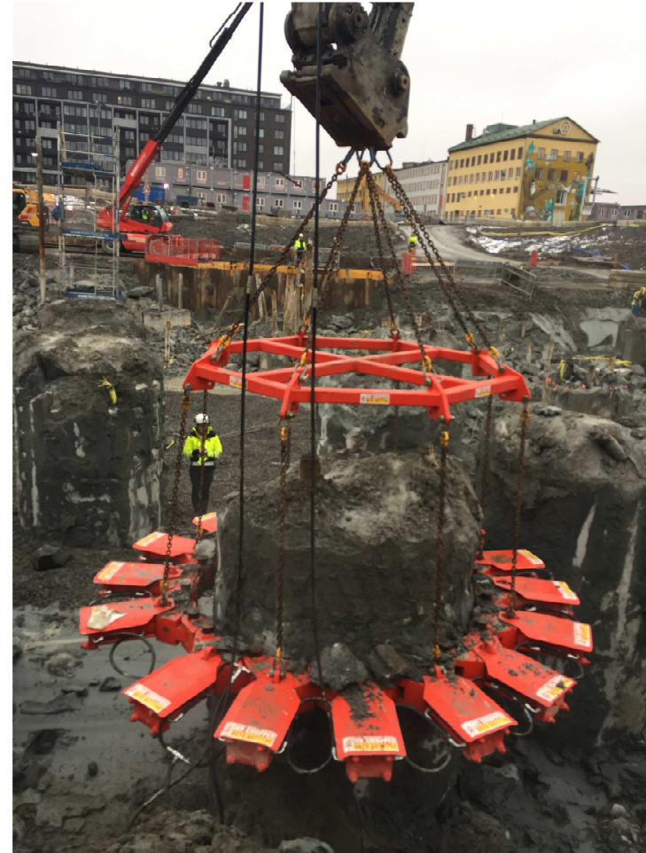
Pile Cap Removal with Cropper and/or the Elliott Pile Breaking Method
