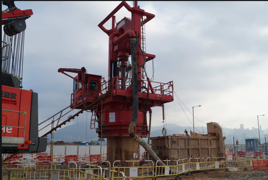
Pile Top Drill Rigs with Reverse Circulation System (RCD) Wirth 818 – vridmoment 180kNm, tryckkraft 800kN
