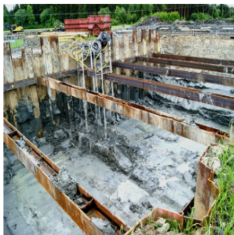
4. Schakt 4.5 m Test 2
