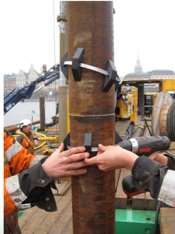
Mounting of pipe clamps
