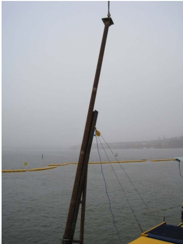
Lifting of steel core
