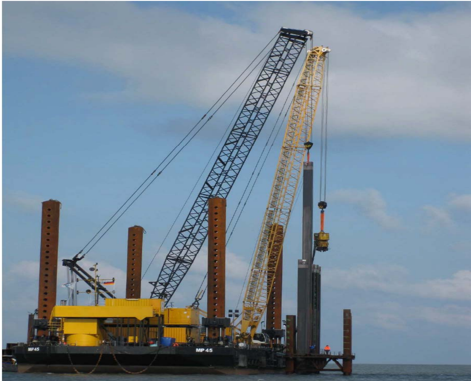
Photo 4: Example of a driving template mounted on pontoon MP 45
