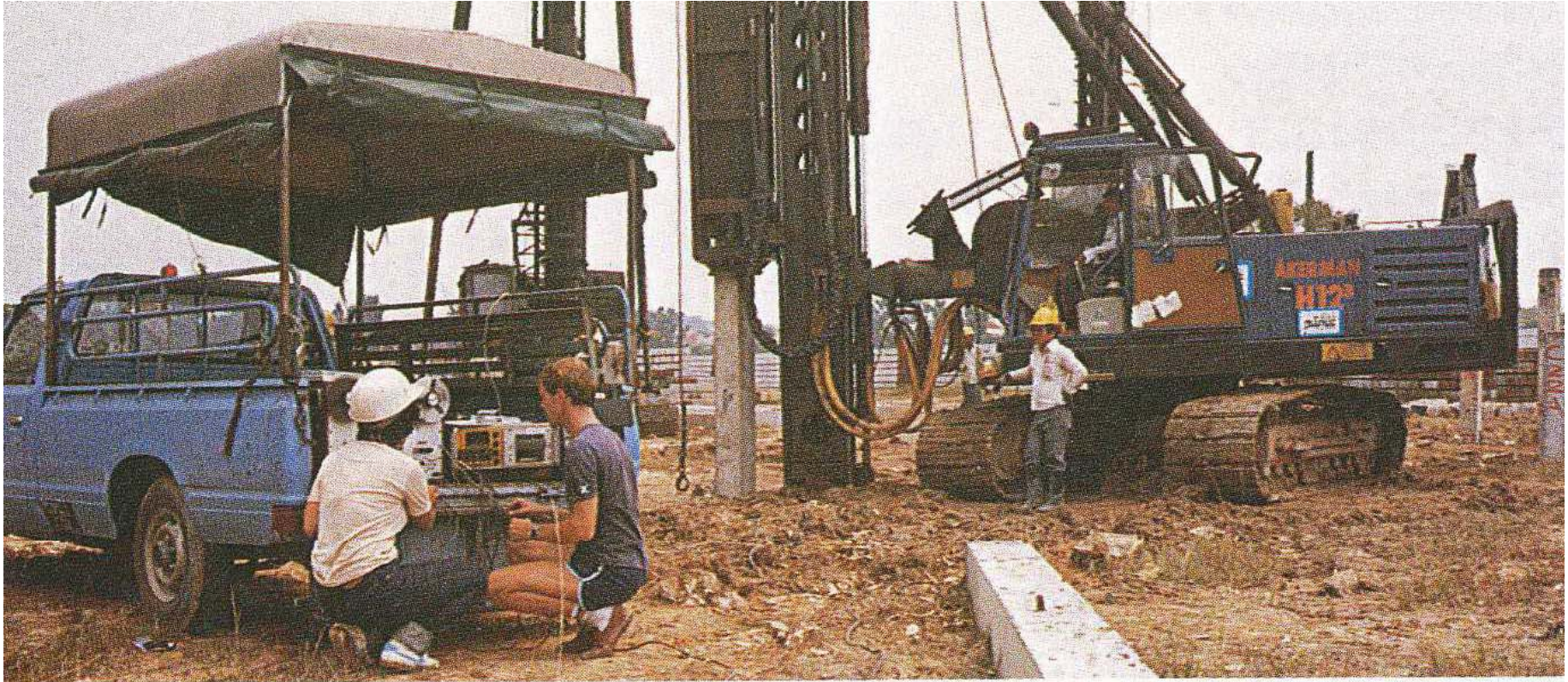
Testing of piles at Mandarin Gardens, Singapore.
